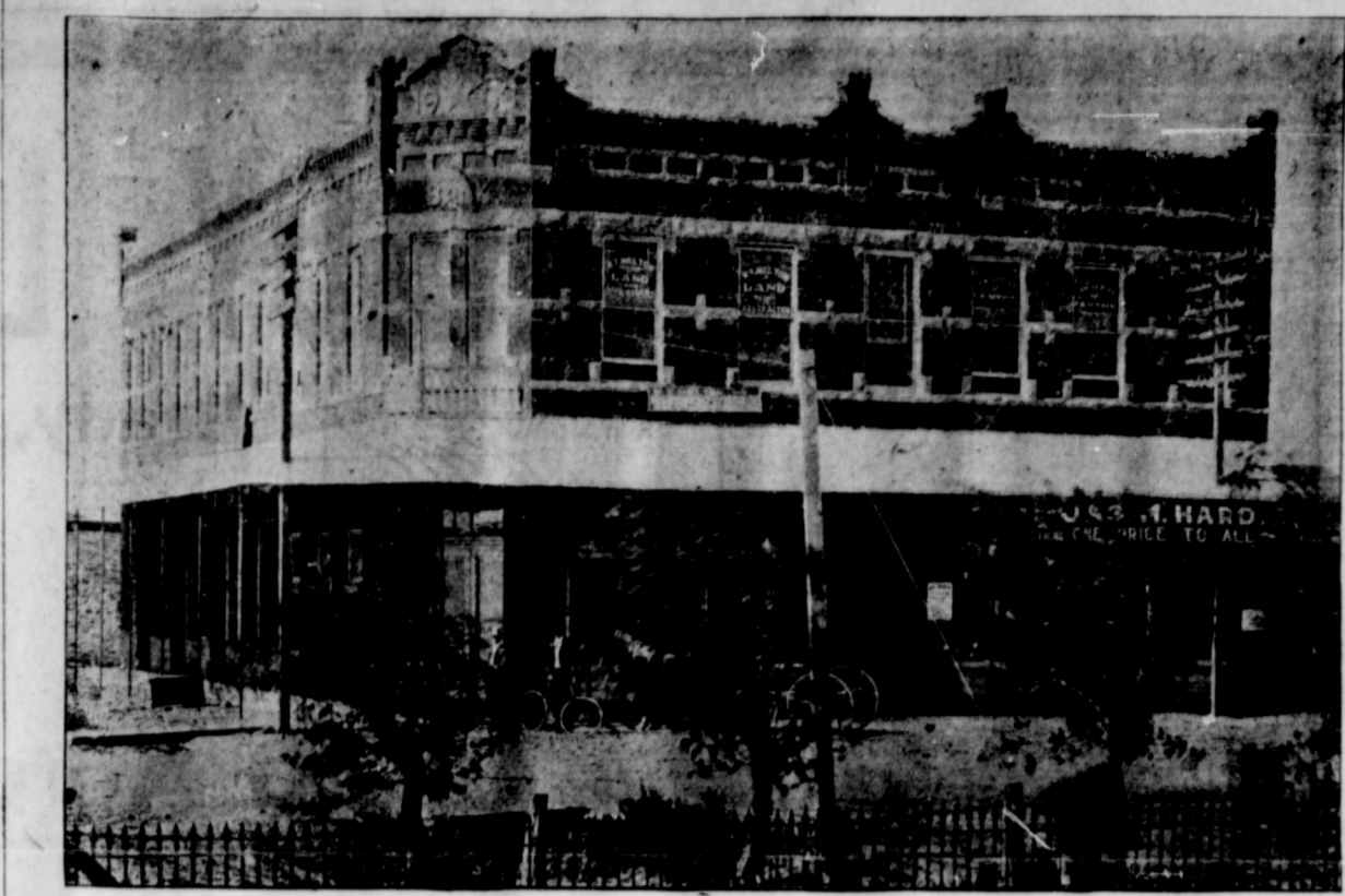
COMMERCIAL NATIONAL BANK BUILDING
