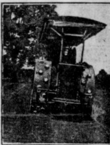
ROLLER WITH "SPUDS" TO COMPACT EARTH ROAD.
