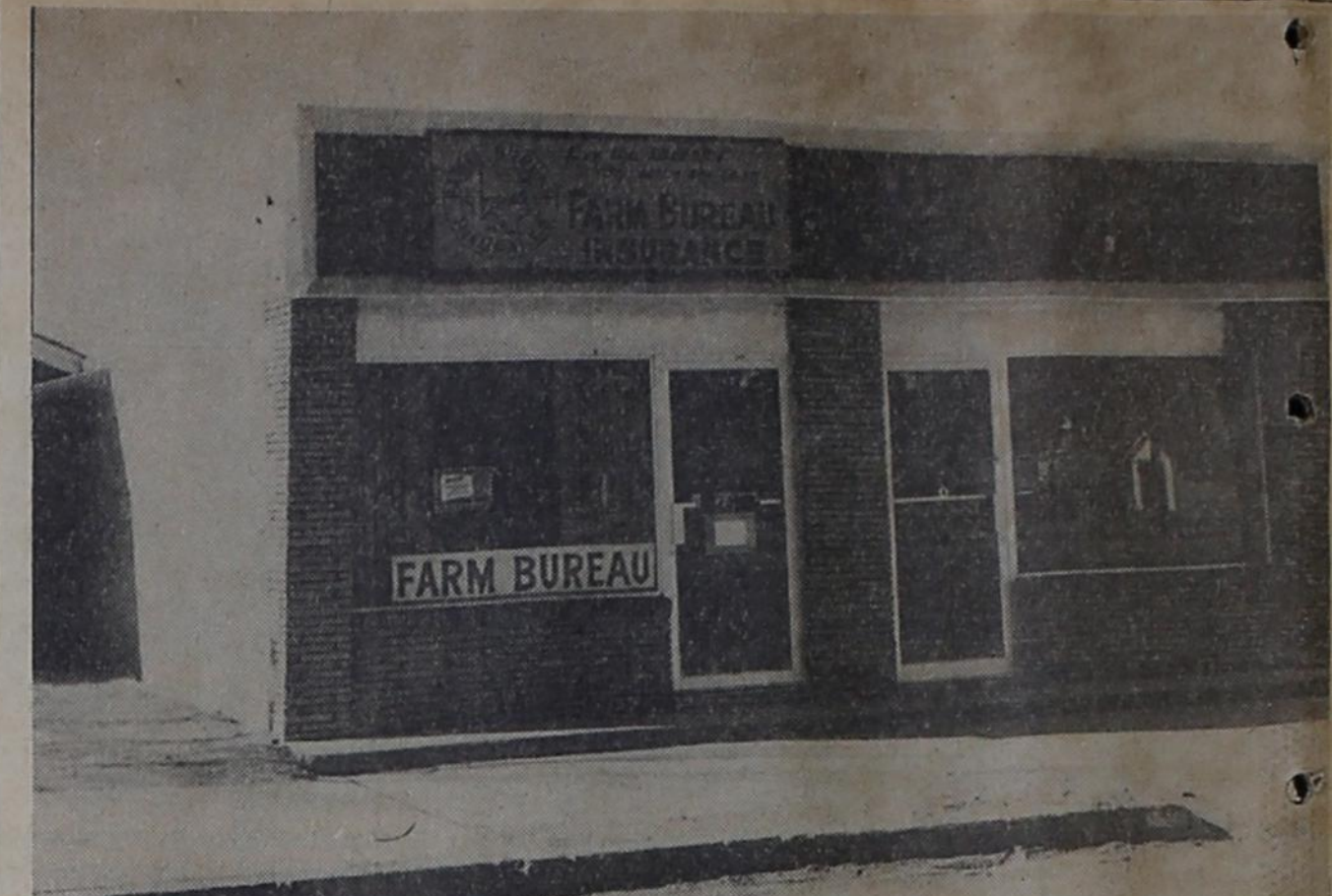
NEW HOME of the Parmer County Farm Bureau is this attractive office building in Friona. It was occupied by the organization and Service Agent Raymond Euler two weeks ago. Bill Garrett, Farwell, is contractor.
