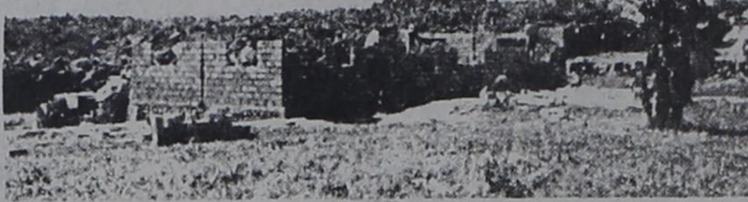
Shown is the girls dormitory being built in Guatemala.
