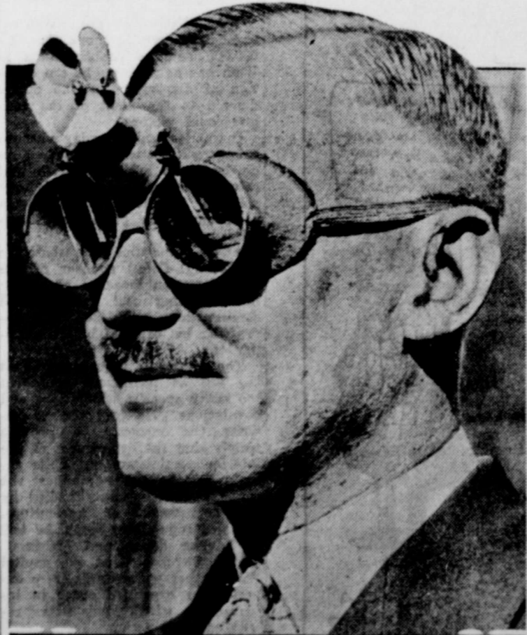
This is L. A. V. Davoren of England wearing a pair of the "rain goggles" that he has invented. They are fitted with windshield wipers which are driven by an exterior air fan that comes into operation when the motorist is traveling at a speed of fifteen miles an hour or upwards.
