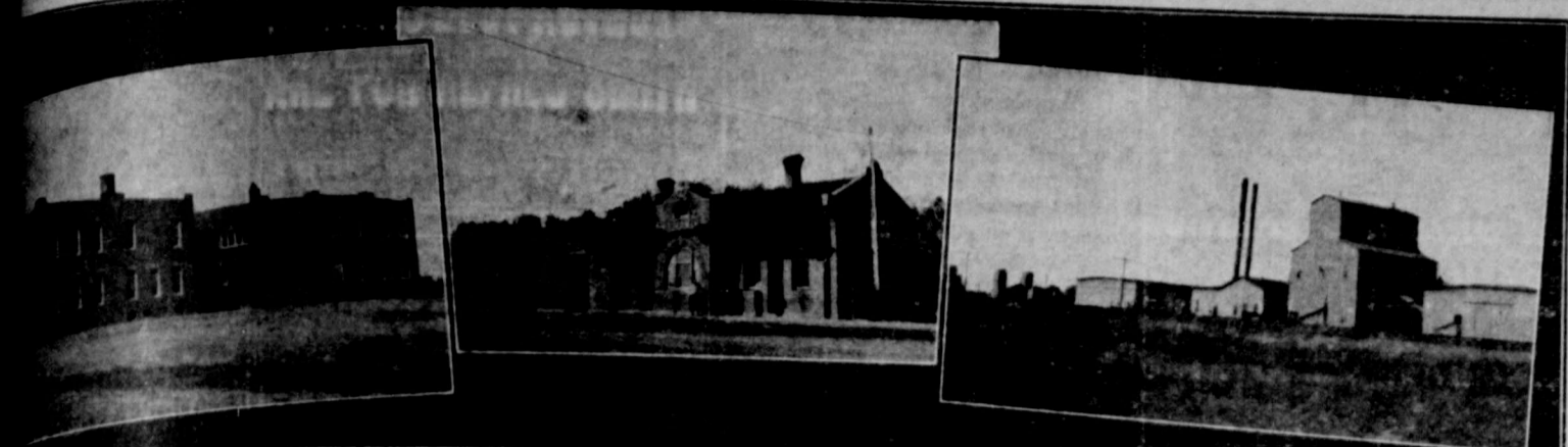
High School Building A. T. & S. F. Depot, Hagerman Pecos Valley Alfalfa Mill
