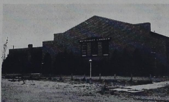
Oklahoma Lane Methodist Church
