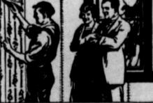
rock - made of gypsum plaster-with Sheetrock Finisher applied at the joints, you can make flat, smooth-surfaced permanentwallsand ceilings.
