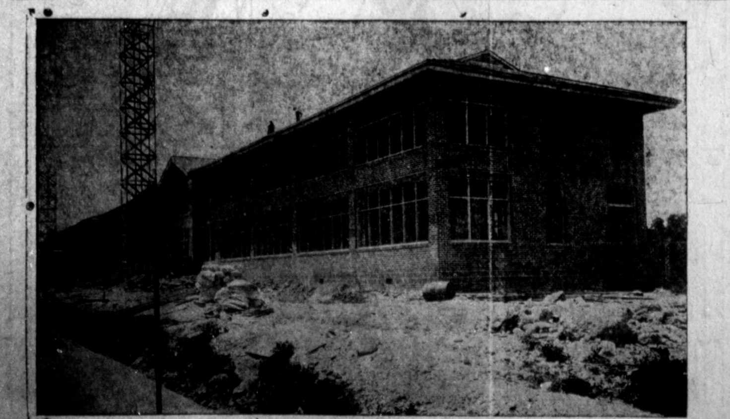
One of the Five Two-Story Ward Buildings, American Legion Memorial Sanatorium
