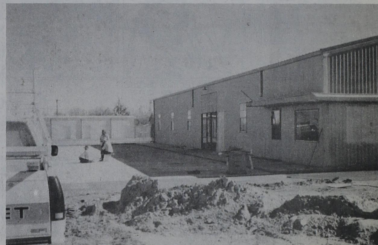
GETTIN' READY FOR BUSINESS... West Texas Rural Telephone Cooperative, Inc., parent company of Friona Communications, is busy remodeling the former Porter building on Highway 60. Workers are paving a new parking lot on the north side for the main entrance to the local business office. WTRTC plans to offer telephone and cable service to Friona. No date was given for completion of the building. (Ron Carr Photo)
