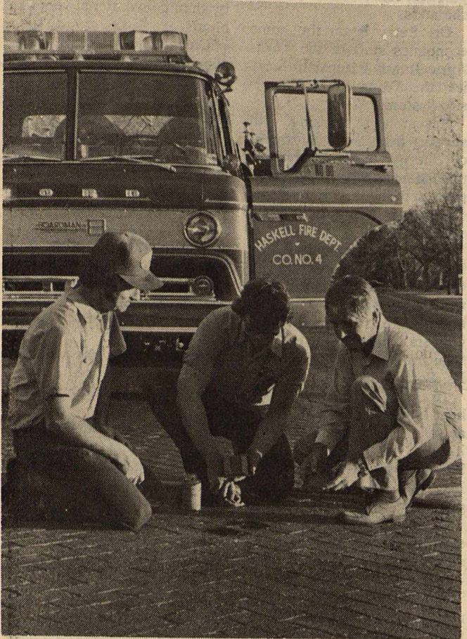
INSTALLING HYDRANT MARKERS
