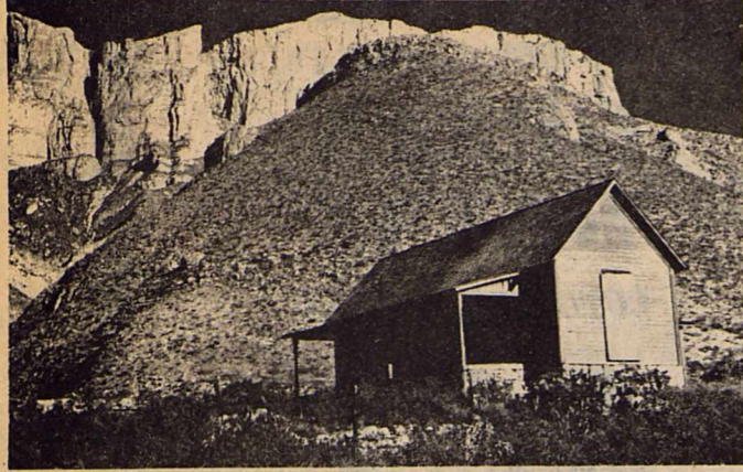
The Williams Ranch House, 4000 feet below Guadalupe Peak on the west side of Guadalupe Mountains National Park, is a stark reminder of the loneliness of old longhorn ranching days. Built in 1908 by Robert Belcher for his new bride, the lumber was hauled by mule train from Van Horn. The bride stayed one night, then went back home. TTDA Photo by Michael Murphy
