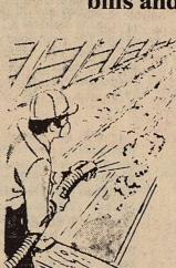
Blown-in Solar Therm insulation
