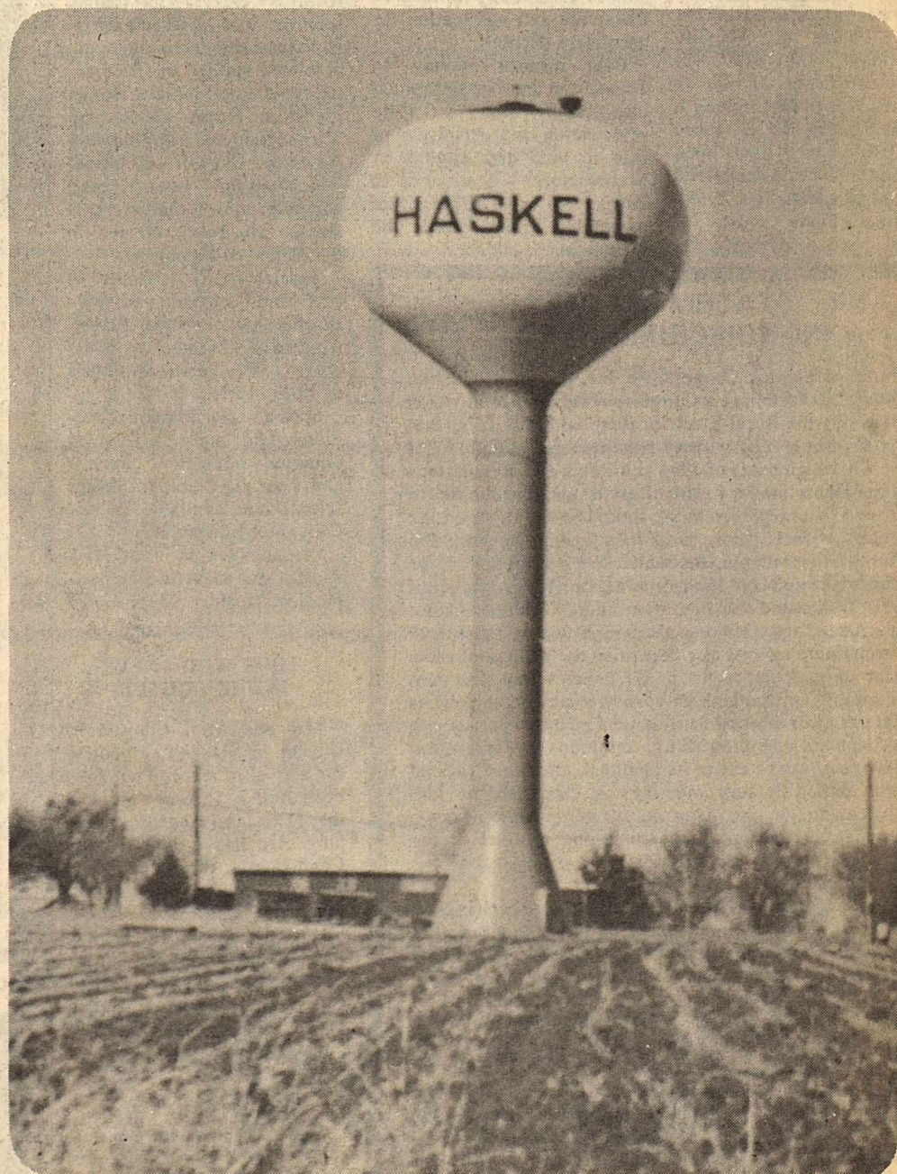
COMPLETED —The new water tower located in the north west part of Haskell is ready for water. The new storage tank has a capacity of 250,000 gallons and will bring the city's total to 820,000. Haskell needed the new storage as they were short of storage. The cost of the tank is $132,000 plus another $25,000 for extra lines. (Photo by W. E. Wooten)
