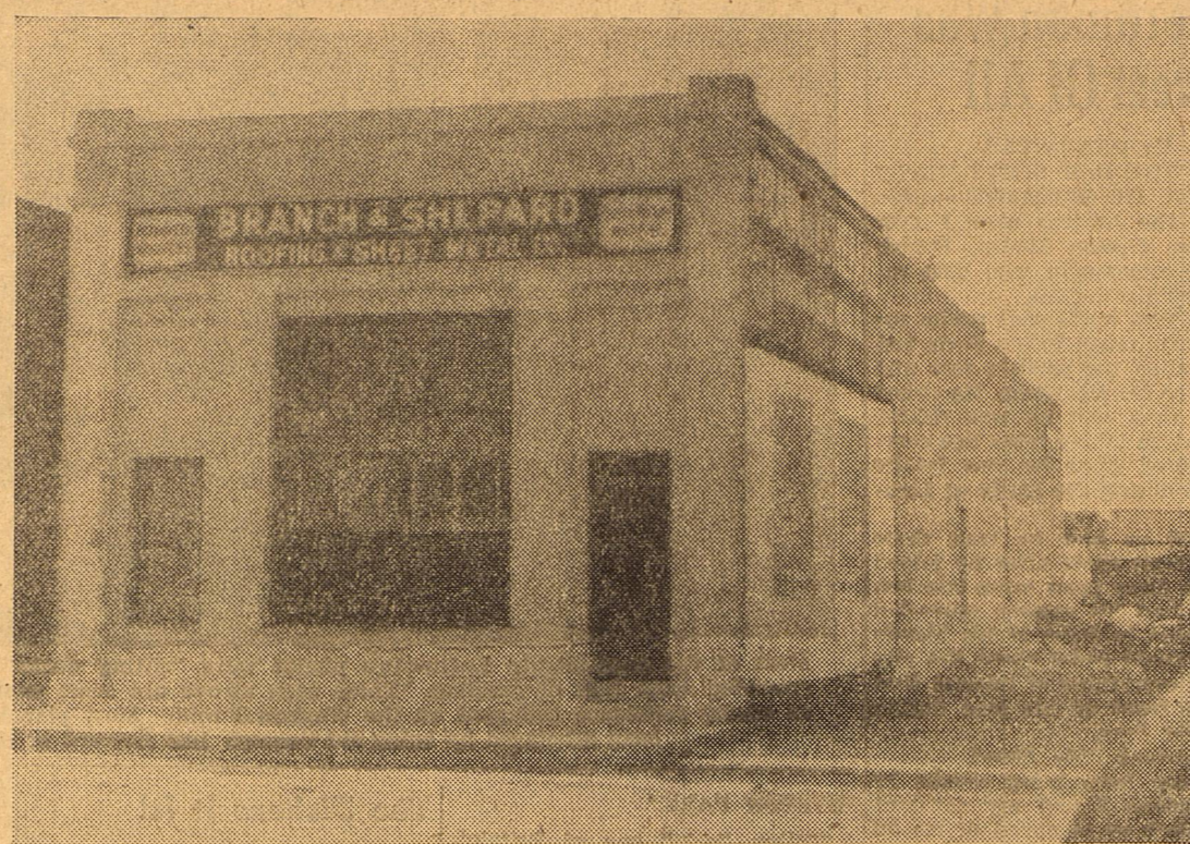
The Branch & Shepard Roofing Co. is owned by D. Branch and C. H. Shepard. The concern has been doing business in Midland since May, 1939, and in that time has solved the roofing problems of many Midland home owners.
