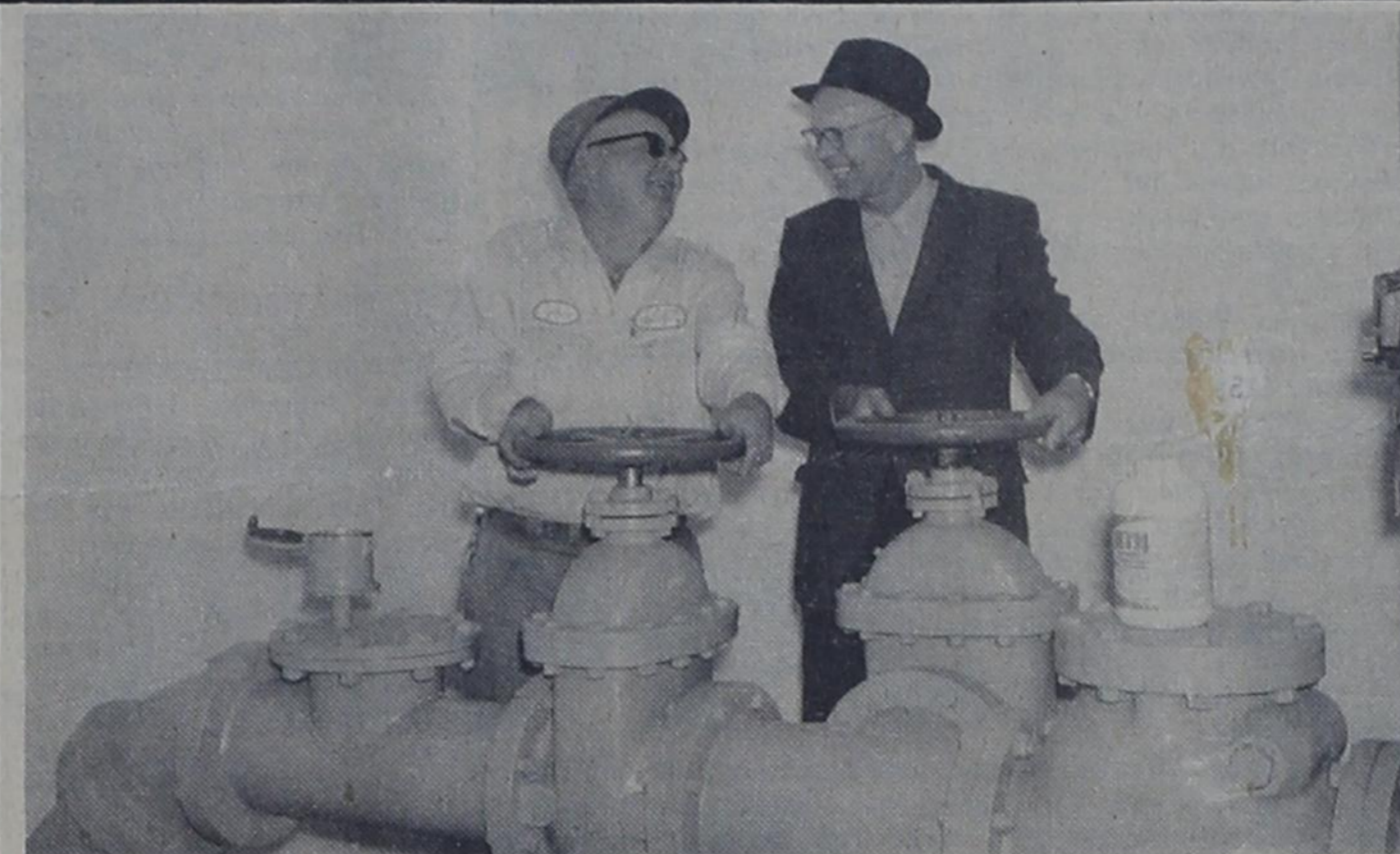
TURNING WATER ON -- Bovina got a new supply of water Friday afternoon when John Wilson, city water superintendent, and Ralph Douglas of Muleshoe, engineer, turned on the pumps of the new 700-gallon a minute well on Ninth Street. At this rate, it takes seven hours to fill the new 300,000 gallon storage tank.
