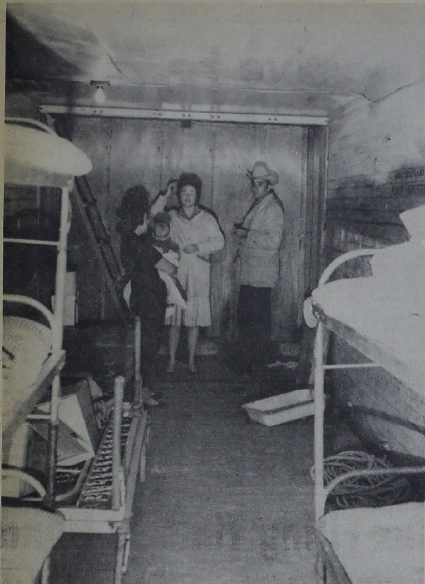
PASSAGE TO SAFETY . . . Mrs. Dean Jones leads the way through the tunnel from the cellar on the Partin Austin farm to the buried box car which is being prepared for a fallout shelter. The refrigerated car is one of the methods used to prepare the shelter for large groups or with adequate living area. Miss Ettie Musil, County home demonstration agent, follows Mrs. Jones with her son, Kyle, on a conducted tour of the installation.
