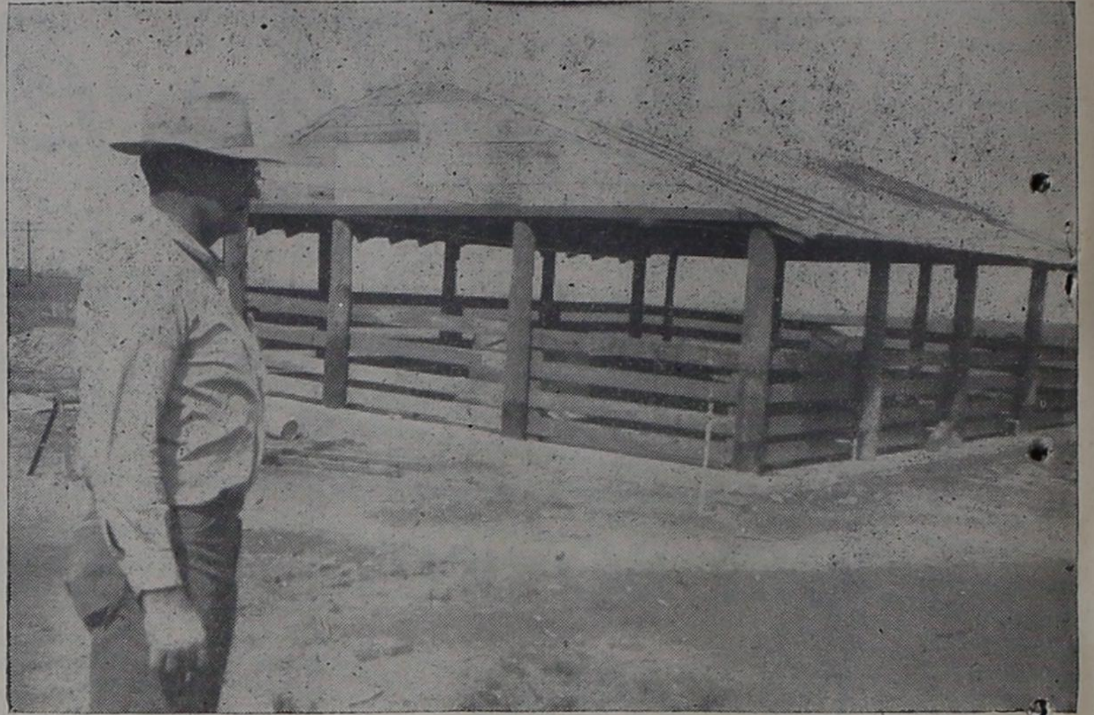
FANCY PIGHOUSE — Doyle Cummings shows what a modern-day "pig parlor" looks like from the outside. The open construction provides good ventilation, yet the pigs are protected from the weather.
