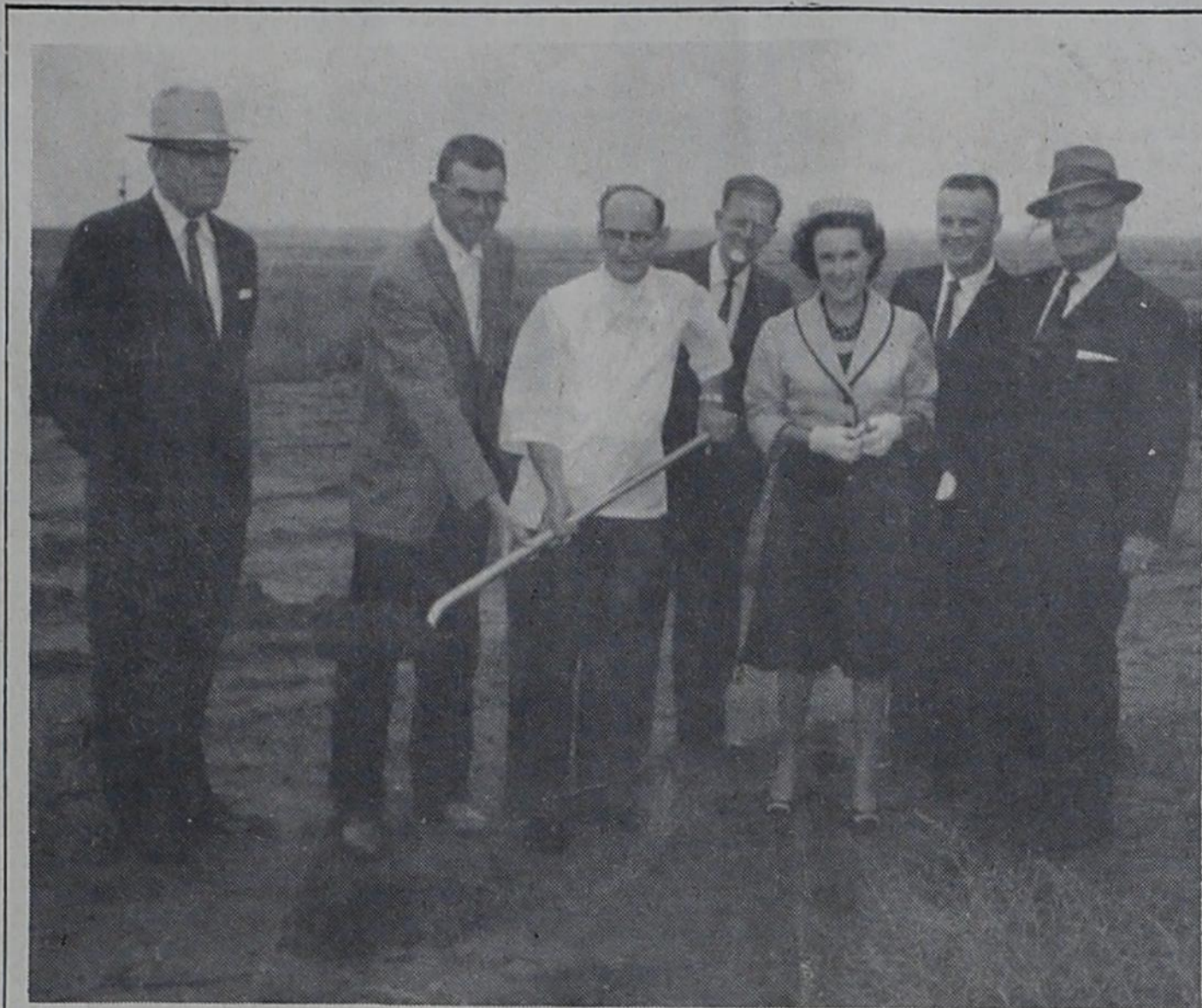
HOUSING DEVELOPMENT GROUND BREAKING--City of Bovina Mayor Emmett Tabor, center, and Chamber of Commerce Manager-Secretary Jack McCracken, second from left, use a golden shovel to scoop first dirt from first house foundation in Ridgelea, Bovina's new housing development. Construction on initial house began Monday. Looking on at the ground breaking are Warren Embree, president of First National Bank, left; Bill Christian, developer of the area, behind Tabor; Mrs. Archie Castleberry, vice president and director of First National Bank; Robert Hopkins of Roswell; and Archie Castleberry, of Amarillo right, a director of First National.
