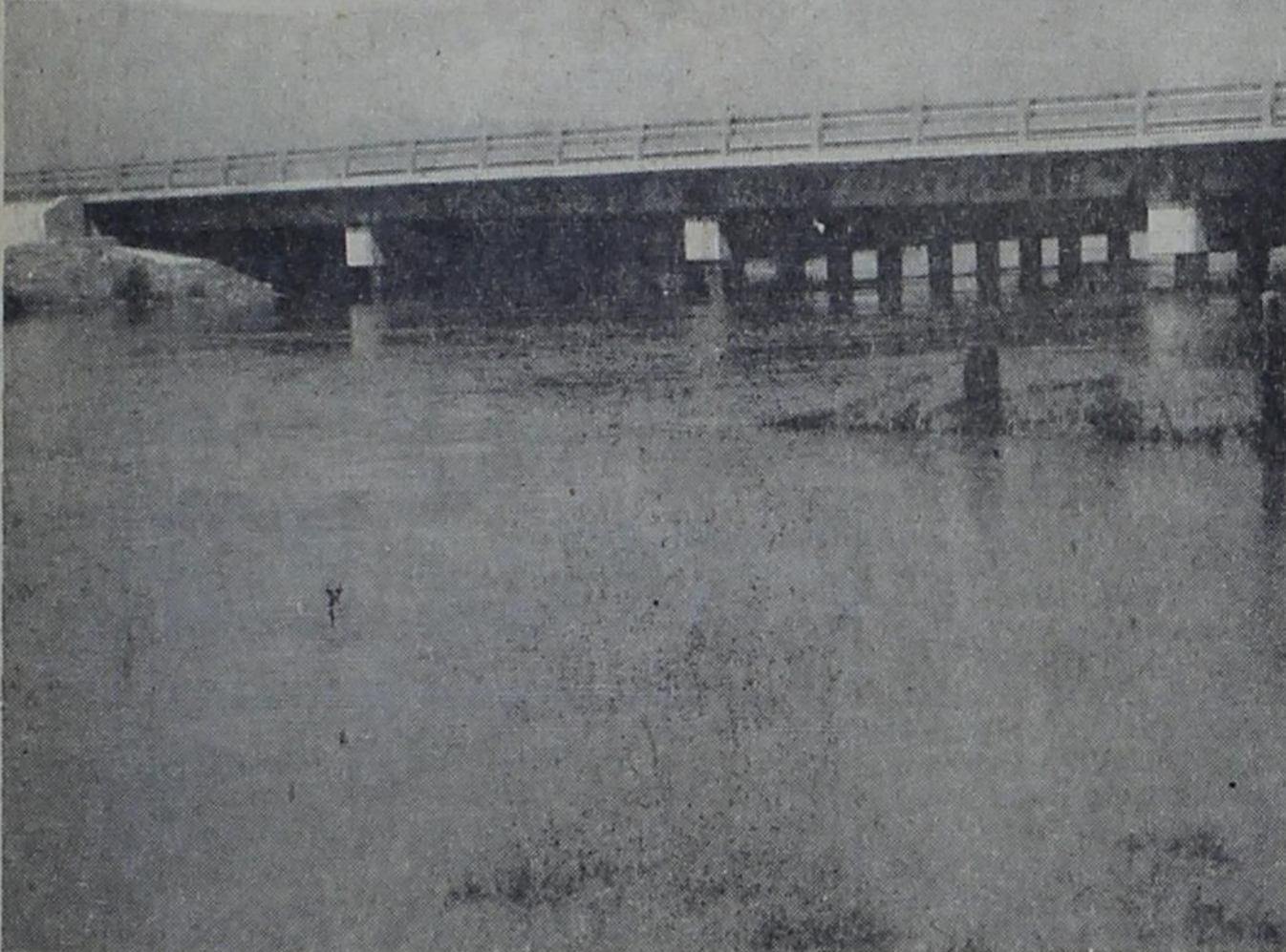
LOTS OF WATER was running under this bridge on Running Water Draw between Bovina and Farwell. This is the fastest the water has been sweeping down the draw in many years.
