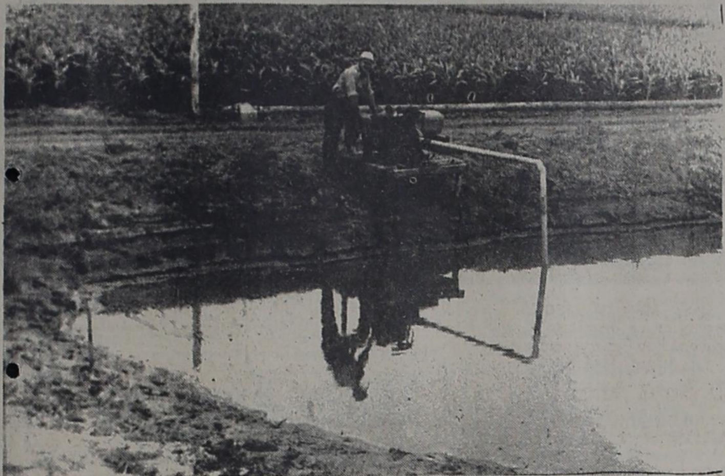
WATER SAVER --This is the system A. J. Reznick, whose farm is north of Friona, has installed to save "tail water" on a half section of his farm. Water is caught in the pit and pumped across the road into an underground tile system.
