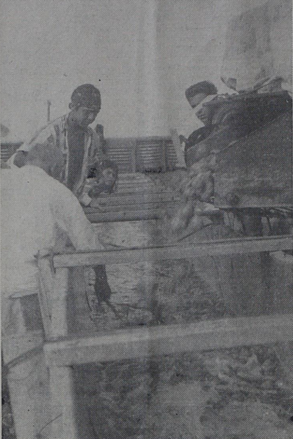
Potatoes fresh from the field of John Hood are dumped into a trough filled with rushing water, where sand, vines and field debris are separated from the spuds before they are carried into the Gregory Produce shed at Lariat.
