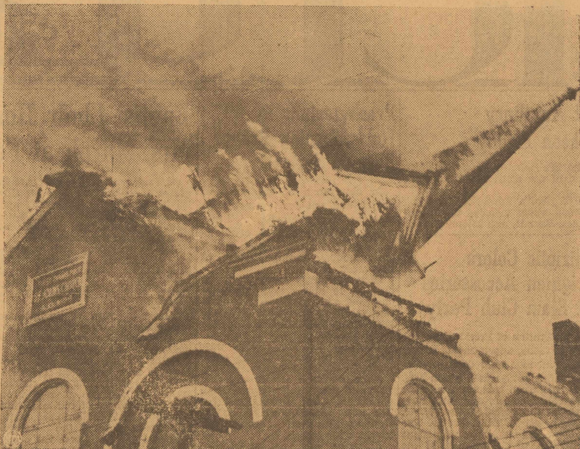
Into the church interior crashes the flaming steeple of venerable St. John's Evangelical Protestant Church at Newport, Ky. Damage was estimated at $75,000.
