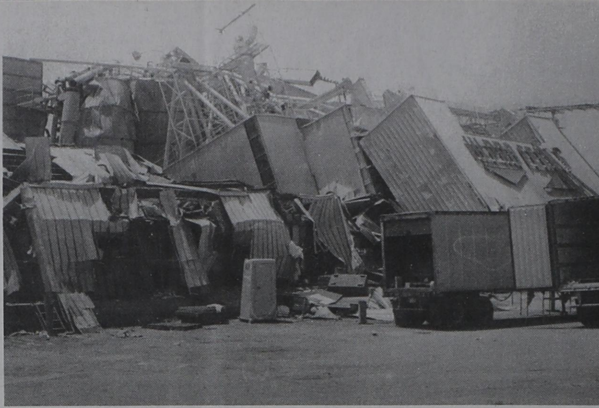
HI-PRO DAMAGE..... An example of the devastating damage that was sustained by Hi-Pro Feeds in Friona last Friday evening is shown in the above photo. Damage to business buildings alone topped $25 million, according to a Friona city official. For a special issue of "Tornado 95," come by the Bovina Blade office on Monday.
