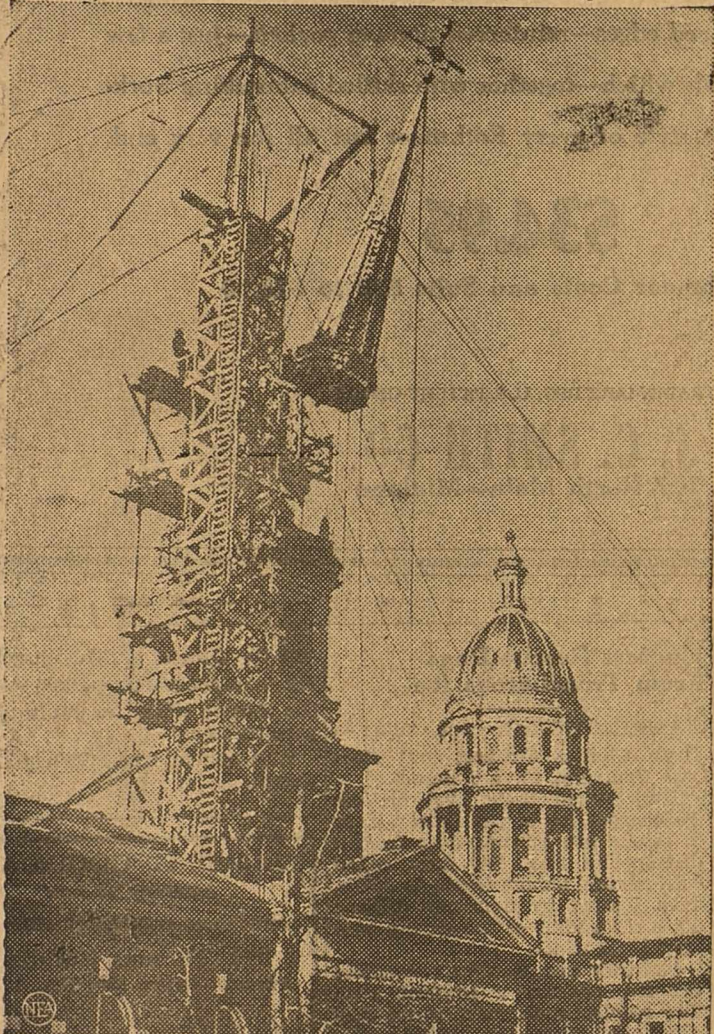
The task of elevating this church in Denver was not altogether spiritual—as this striking photo indicates. To erect its graceful 160-foot steeple, workmen first assembled the spire on the ground and then hoisted it into place by complicated derrick maneuvers. In the background of the church glitters the dome of the Colorado State Capitol.
