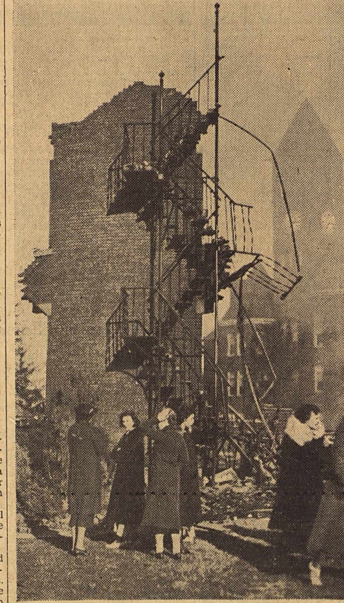
Strangely alone after the building to which it was attached had fallen before flames, this fire escape was one of the few parts of the Slippery Rock Normal School, Slippery Rock, Pa., that was left standing after the fire destroyed the structure. Girl students with coats over pajamas stroll slowly by and in the background, through the haze of smoke, stands a steeple with the clocks gleaming faintly.
