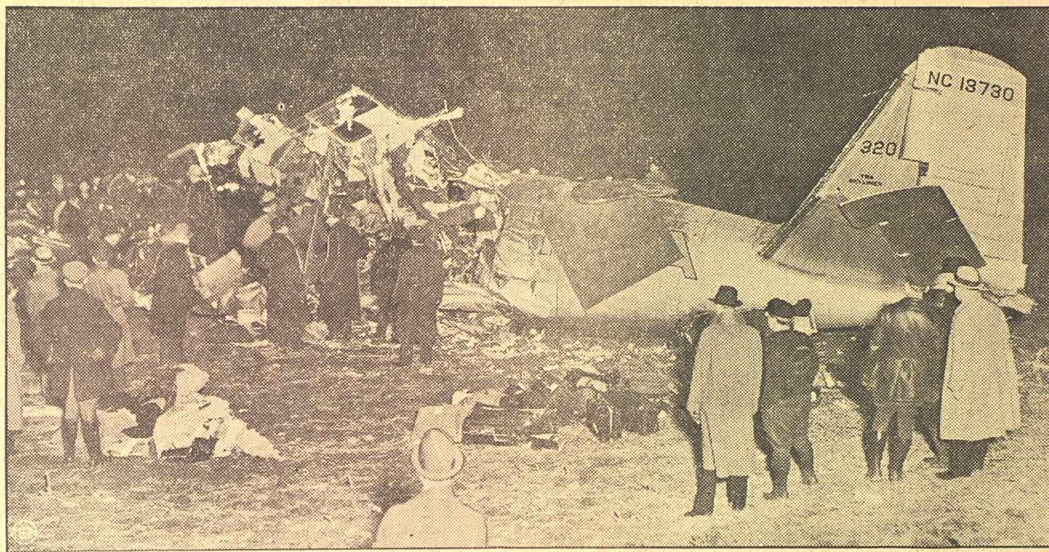
Five minutes earlier, it was a giant flying machine. Here it is a huge mass of wreckage with some of the 13 victims, killed when the TWA liner crashed five miles southwest of the Pittsburgh airport, still in the crushed fuselage. Ice on the wings was one suggested cause for the mystery crash which occurred just before the pilot was to make his scheduled landing after a flight from Newark. The plane, which had been working perfectly, apparently fell several hundred feet. Notice how baggage on the ground is split open. The ship did not catch fire. It was the seventh air crash in three months, sending the death total to more than 50.
