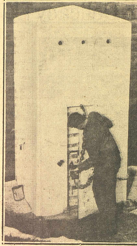
It may be midday, but darkness is falling for the prisoner inside as the outer door, which shuts out light, is swung shut. It will be double locked and the chain will be drawn around as a triple safeguard against escape.
