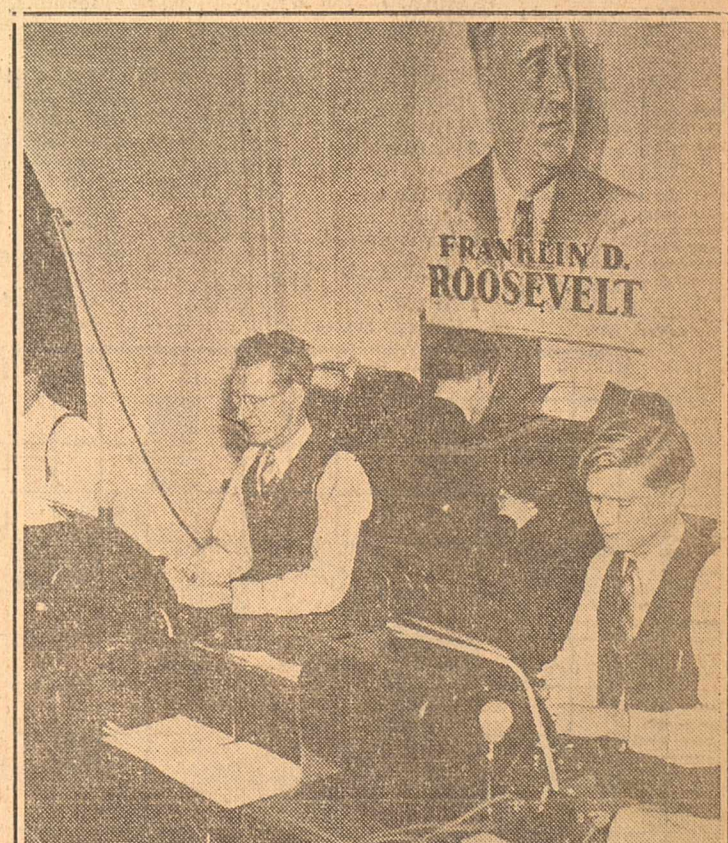
Acting on orders of President Roosevelt to give the absolute limit of co-operation for flood relief, the WPA musters its full power of men and equipment in the disaster areas. Washington headquarters keeps in direct contact with local offices through the corps of ticker operators sending and receiving messages above.
