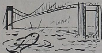
THE VERRAZANO-NARROWS BRIDGE, BETWEEN STATEN ISLAND AND BROOKLYN, NEW YORK, HAS A SUSPENSION SPAN OF 4,260 FEET, LONGEST IN THE WORLD, AND EXCEEDED THE GOLDEN GATE BRIDGE OF SAN FRANCISCO BY 60 FEET.
