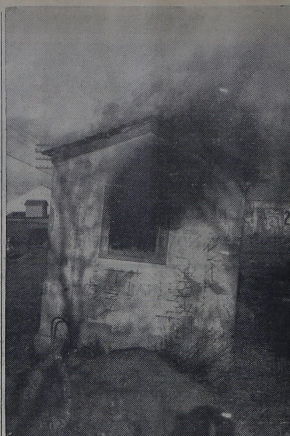
THE END OF AN ERA —Fire, origin unknown, wiped this building, one of the few outdoor toilets left in Bovina, off the slate Monday afternoon. The unsightly structure was located in the alley between the railroad and North Street. The fire department did not come to the scene, feeling that the flames were bringing about good riddance. One North Street businessman commented, "I don't know who started it, but I wish I did. I'd like to buy him a malt."
