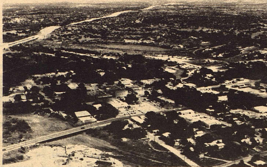
1,000 feet over Sonora, Texas-looking northeast
