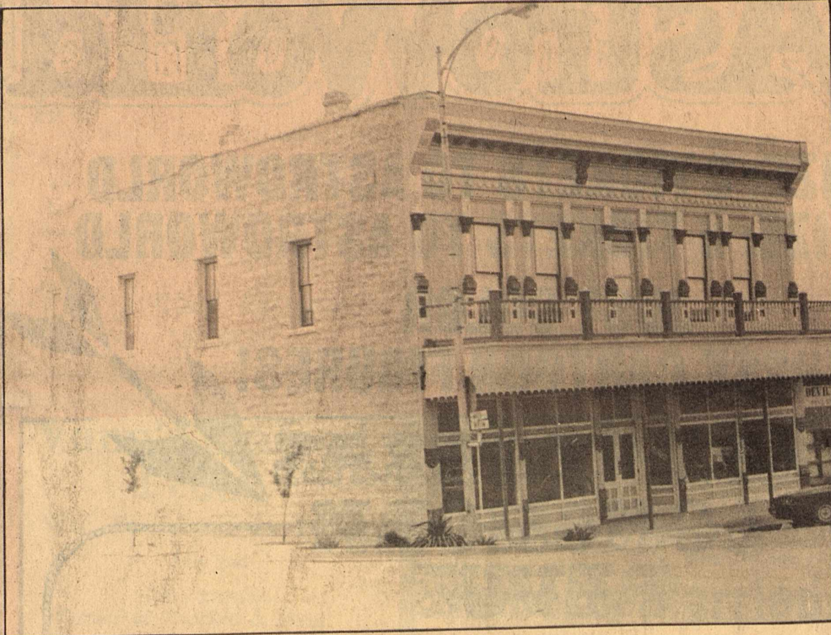
Old Mercantile Building Designated Historical Monument (See story, page 7)
