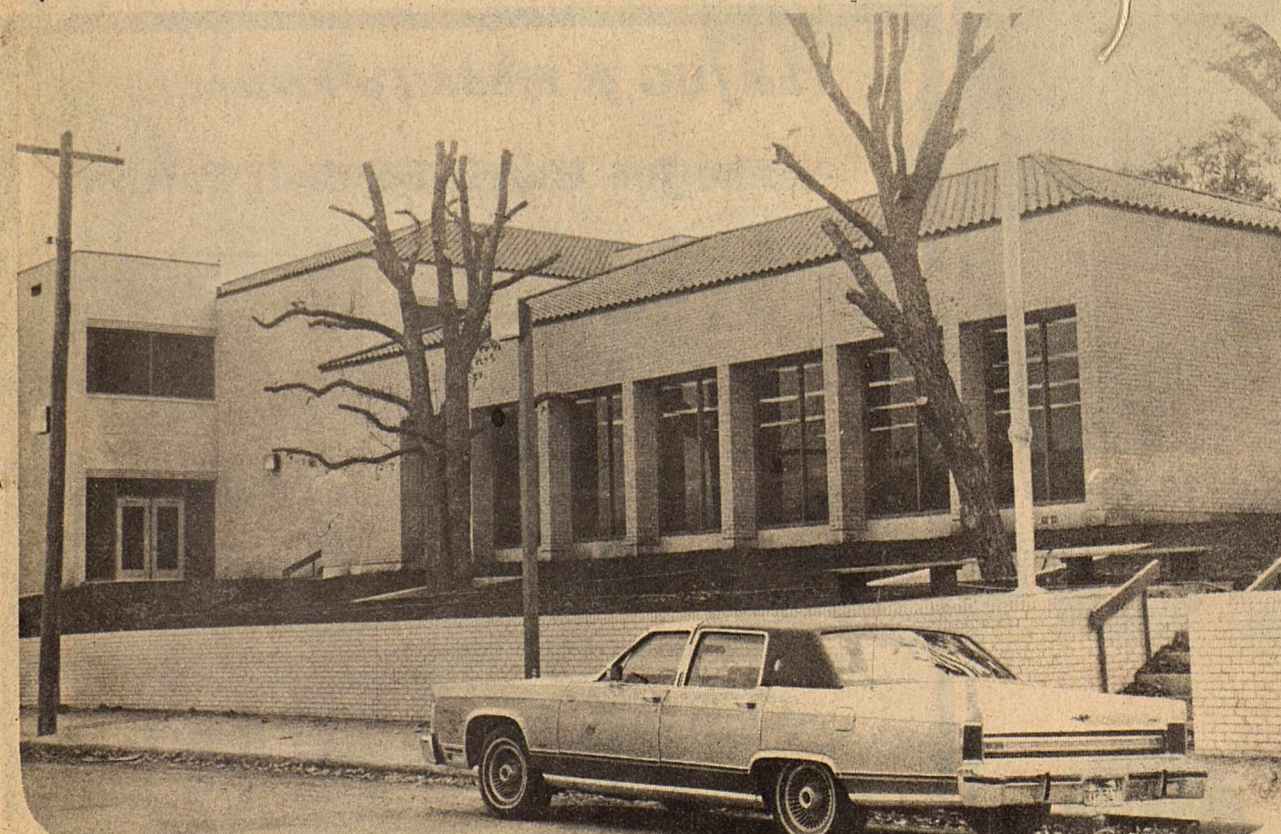
New Junoir High Building Almost Ready !
