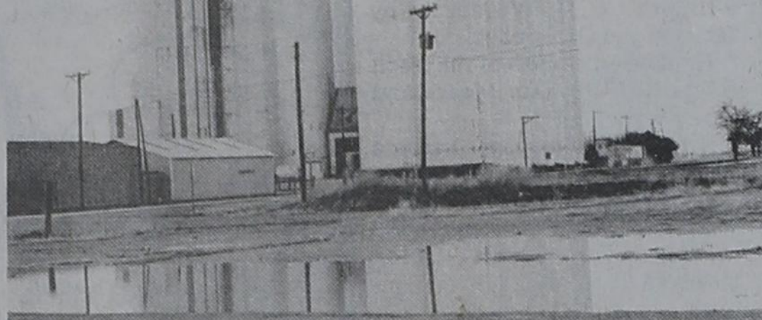
WATER, WATER...A good example of the water that was standing following Monday's rain is this picture, looking east from Third Street.
