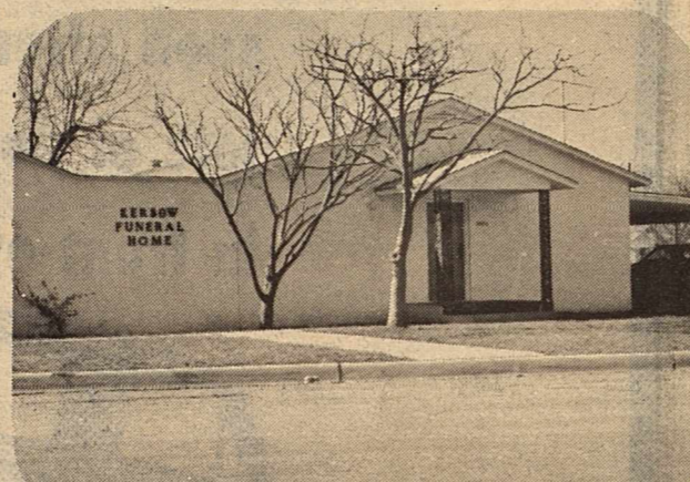
Kerbow Funeral Home has recently been remodeled and a chapel has been added to provide even greater service.
