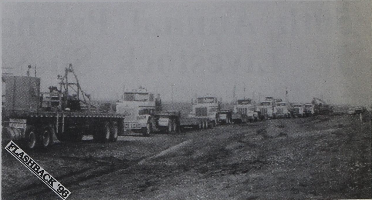
WIDE LOADS..... This convoy of wide horsepower was used to bring the huge track moving cranes in last week as work continues on the Santa Fe Railroad construction.
