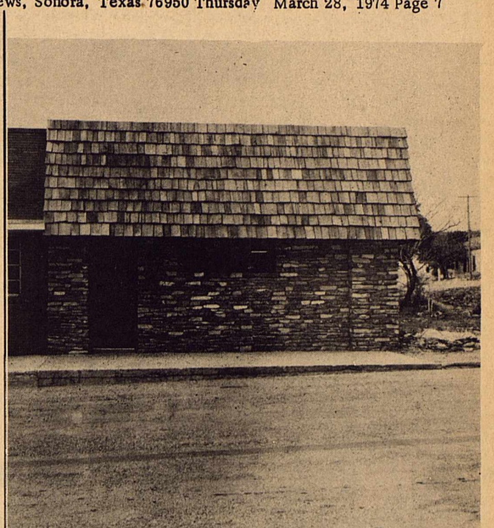
NATIVE ROCK AND cedar shingles provide the finishing touches to the newly renovated office of C. Adam Morris, III, Attorney at Law. The building that once housed the Sonora Men's Store and dry cleaners, operated by Fay and John McClelland, has taken on a complete face lifting with the assistance of King and Sons Ranchette Builders, who did the inside and outside work. Morris also serves as County Attorney, operating from this office instead of the office located in the County Courthouse.
