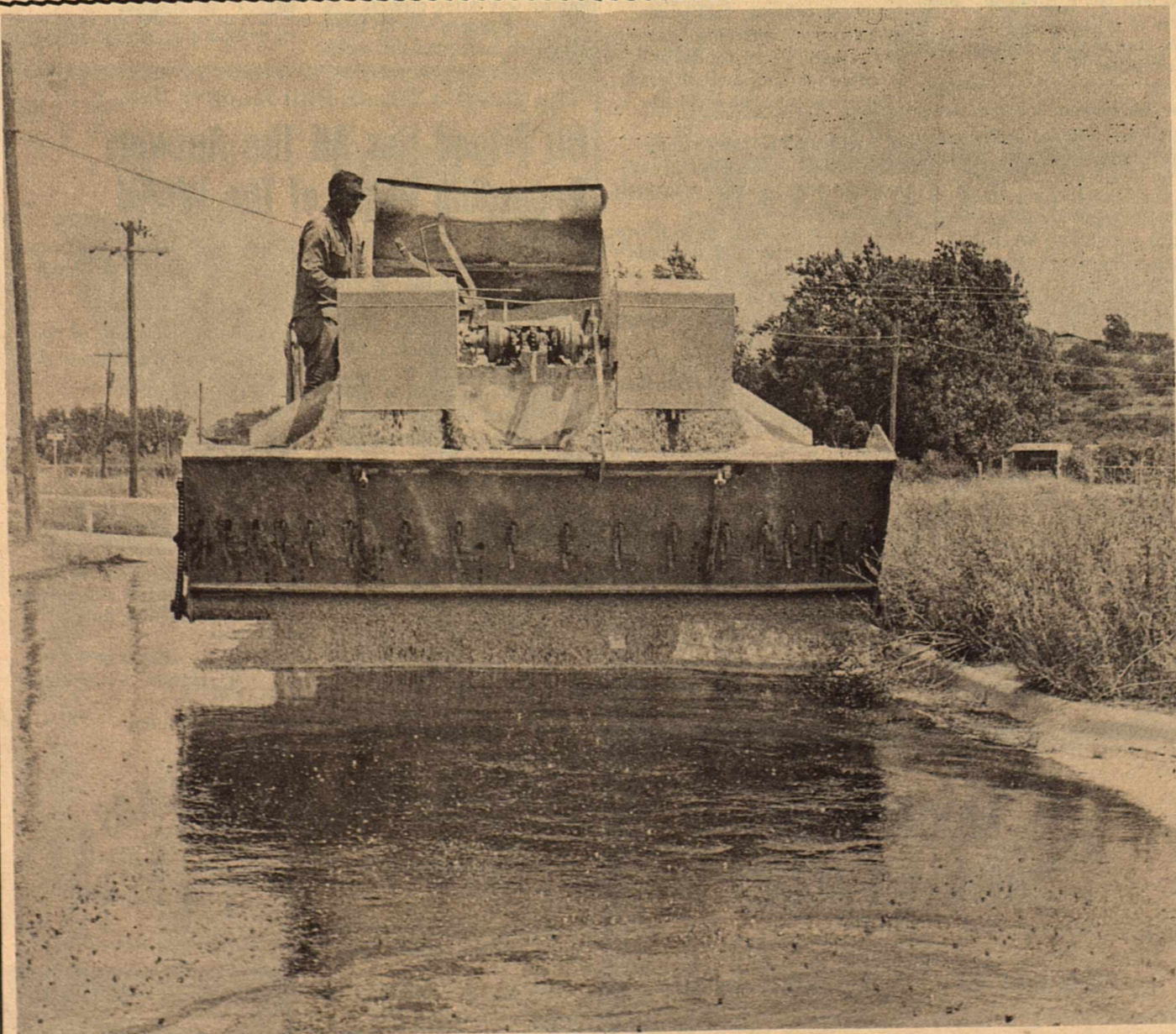
WILSON PAVING COMPANY of San Angelo should complete their seal coat work being done on City streets, this week. City Manager, Alex Binford stated that only streets in most
