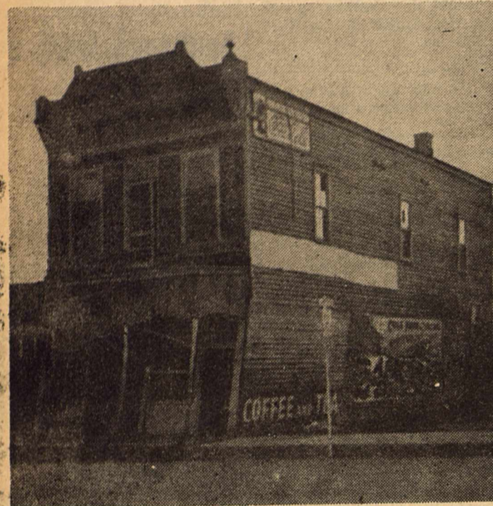
A "LEANING TOWER OF PISA" was once located in Sonora although in somewhat different form than the Italian version. The old Craddock building or "Medical Arts Building" as it was known to many, assumed its leaning position as a result of an explosion in the building.
