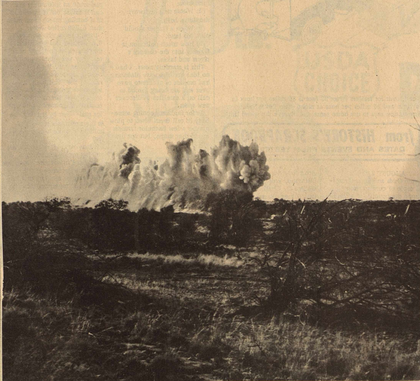
IN ROCKY AREAS IN WEST TEXAS, Oasis Pipe Line Company used a blasting method based on aluminum metal as reaction fuel to blast trenches for the pipe. Rock then is removed from the trench with a backhoe. A minimum covering of three feet
