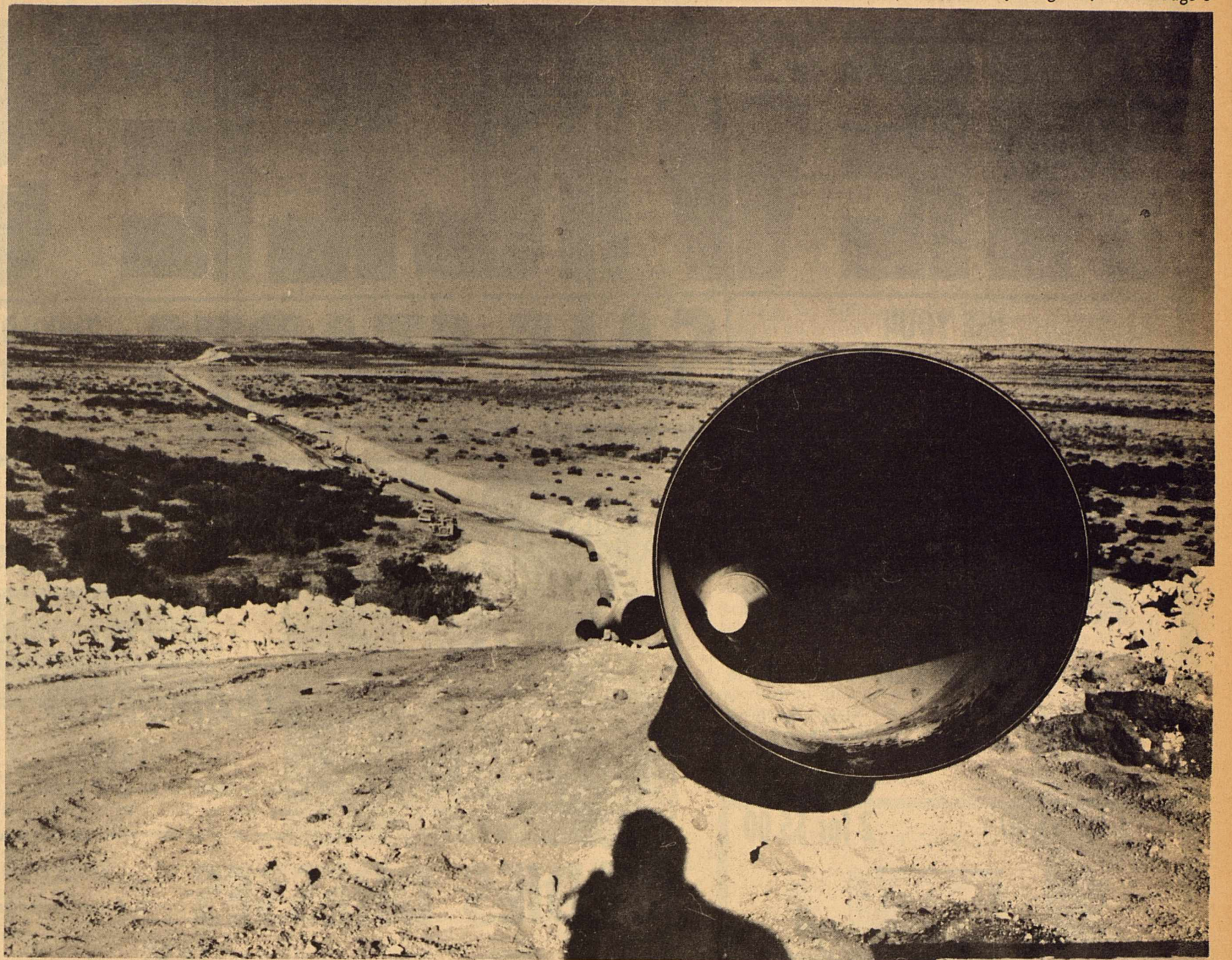
OASIS PIPE LINE COMPANY'S COMPLETED SYSTEM FROM WEST TEXAS to the Houston area will be 508 miles long, approximately the distance from New York to Detroit. The Ozona compressor station is one of six along Oasis
