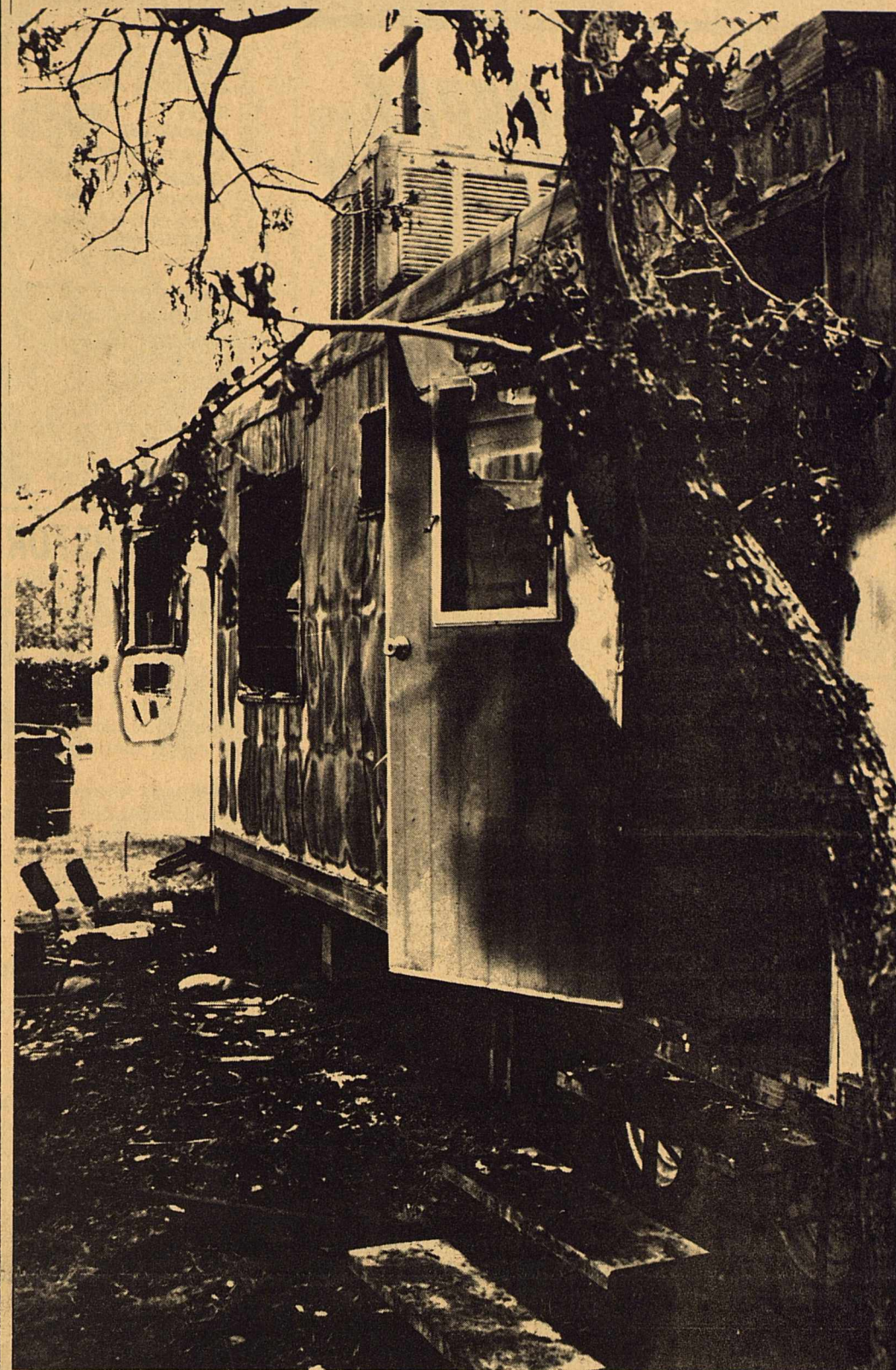
FIRE OF UNDETERMINED origin gutted this trailer house Thursday night while the occupants, Mr. and Mrs. Douglas Woods, were away from home. The trailer belonged to Mr. and Mrs. James Floyd. Contents of the trailer were destroyed completely before the fire was discovered and reported to the fire department.
