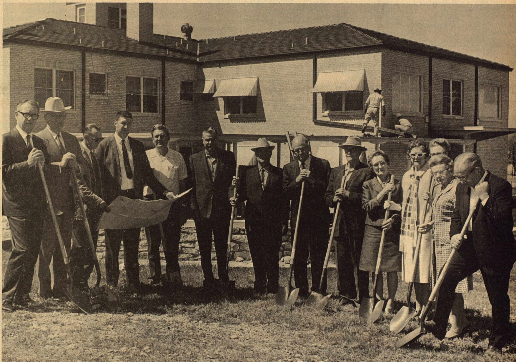
TURNING THE FIRST SPADE OF DIRT Tuesday to signify the beginning of construction on Sonora's new nursing home drew this large group, which includes Hudspeth Memorial Hospital's medical staff, hospital board, administrator and construction superintendent.
