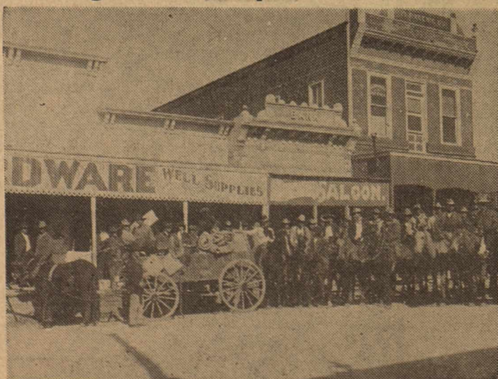
THE BANK SALOON was in fact built in one of the old banks of Sonora that failed. It was owned for a time by Jim Barton. The Craddock Building or the Medical Arts Building is pictured on the right. Evidently this picture was taken before 1911 when an explosion in the Craddock Building gave it a slightly tilted look.
