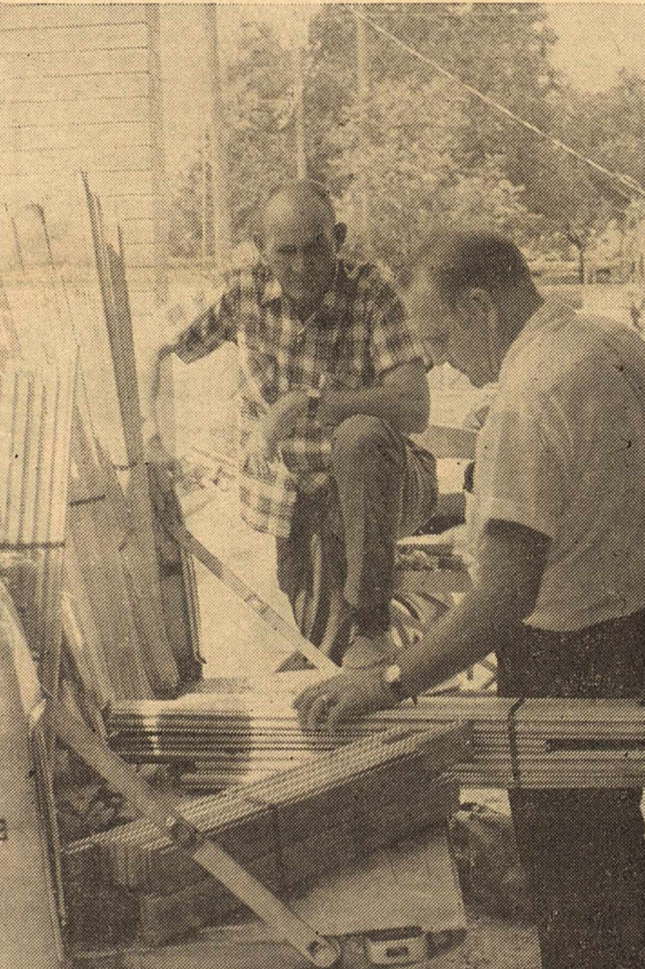
CONSTRUCTION SUPERVISOR RAY DUNLAP and Don Smith inspect a shipment of pre-cut maple flooring material to be used in the gymnasium.
