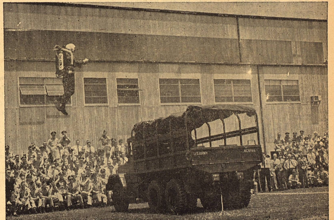
ARMY DEMONSTRATING THE "FLYING BELT." Using the experimental Small Rocket Lift Device (SRLD), believed to be the first portable rocket equipment to carry man in individual controlled free flight, a test engineer soars over a truck during the recent Project Mobility demonstrations at Ft. Eustis, Va. In previous tests, the experimental "flying belt," developed by Bell Aerosystems Co., Buffalo, N. Y. for the U. S. Army Transportation Research Command, has flown at a speed of 20 mph and has made lateral flights of up to 360 feet.
