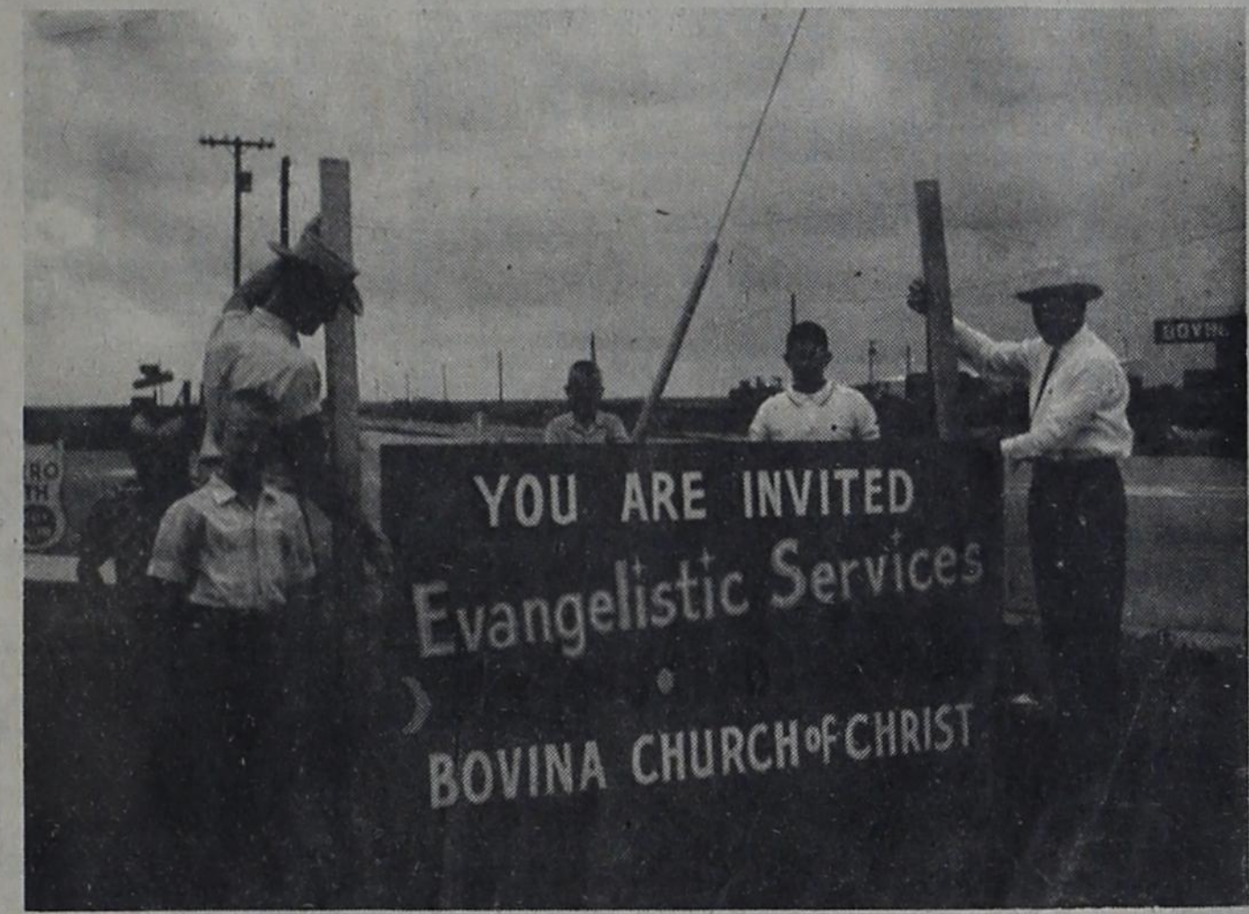
SIGNMEN--Robert Read, at left end of sign, and Buck Ellison, at right, are shown erecting a sign announcing evangelistic services at Bovina Church of Christ this week. The sign, along with others in town, was put up Sunday afternoon. Boys assisting with the work are, left to right, Dennis and Mickey Don Ellison, Tommy Crump and Billy Lynn Marshall.
