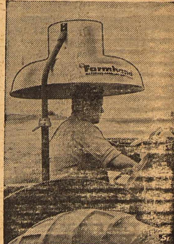
A farmer's inventiveness has resulted in a unique machine which in effect brings air conditioning to operators of tractors and self-propelled combines. No longer is running these machines the hot, dusty job of the past. The unique machine, called the Air-Brella, shades, cools and protects the driver from dust, insects, fumes, sprays and dusting chemicals.
