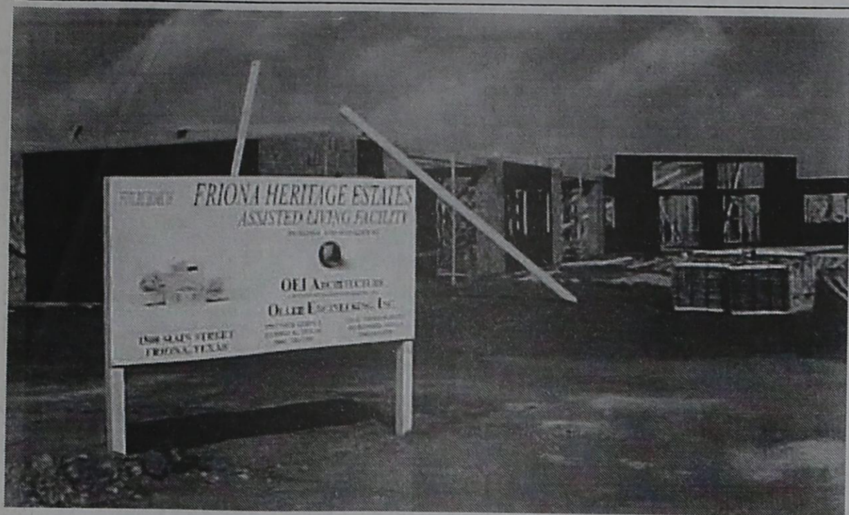
FRAMING WORK is underway on Friona's assisted living complex, "Friona Heritage Estates," giving an idea of what the new facility will look like. Located adjacent to Prairie Acres, the facility has a waiting list that could fill it up when complete. (r. carr)
