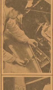
Hudson engineers this year have placed the automobile battery where it is easily accessible, under the hood, as shown in top photo. Below is shown the new 1937 Studebaker door, which its makers claim a child can close with one finger because of new rotary door locks.
